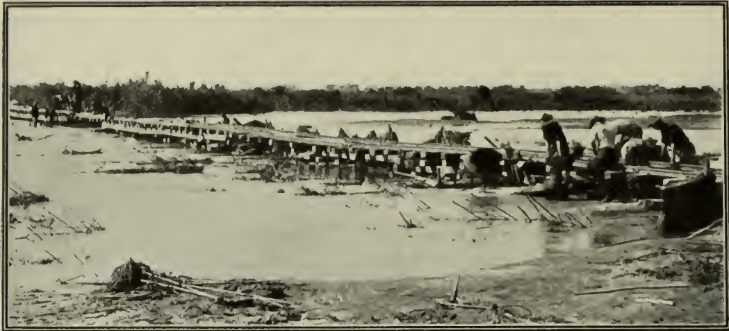
REBUILDING RAILWAY TRESTLE CARRIED AWAY BY A WASHOUT NEAR TARLAC.
